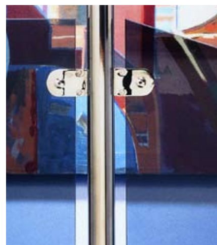
Glass Infill Mounting
