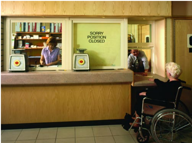
H513 Lowered counter and parcel hatch to provide counter service for wheelchair users.
