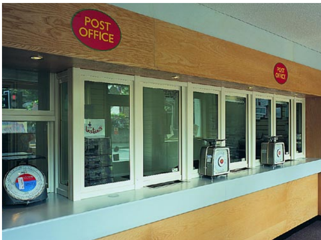
Protection screens meet the Post Offices physical attack and installation requirements.
